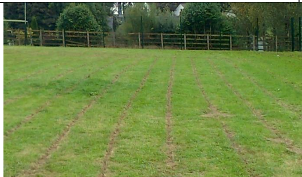
Dripline is usually mechanically inserted 150 -200mm BGL into topsoil when soil depth to limiting condition is sufficient. Finished systems are hardly visible.
