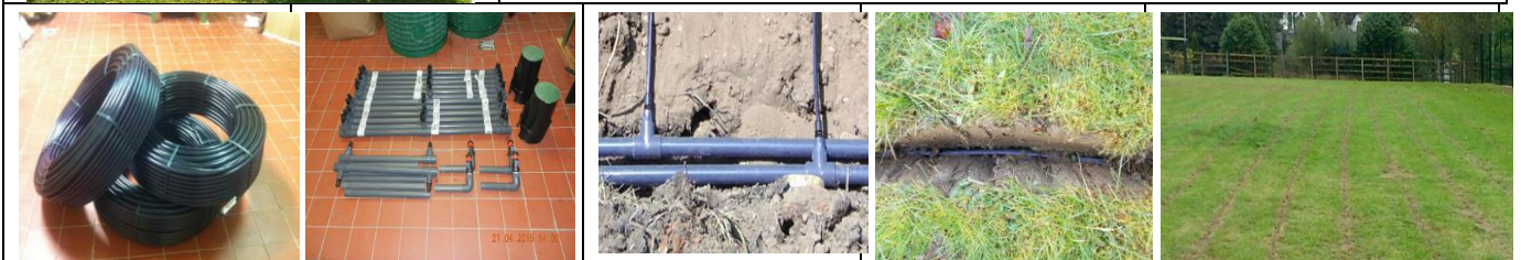
A series of driplines are inserted into the ground and connected to a pump tank and a secondary treatment system
